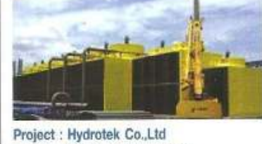
Project : Hydrotek Co., Ltd Model : BKC-S-700 RT x 1 Cells BKC-S-800 RT x 2 Cells BKC-S-1500 RT x 8 Cells
